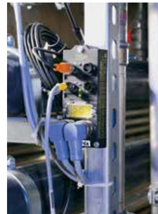
I/O Blocks are located at each system component.
